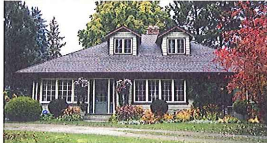
334 Beach Avenue $1,740 (new dormer windows)
